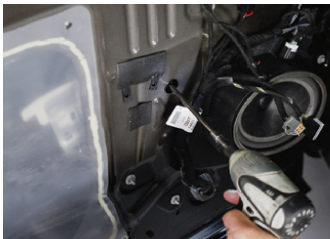
▲ Figure 17. Replacing the front window regulator bolt through the window regulator bolt access hole
