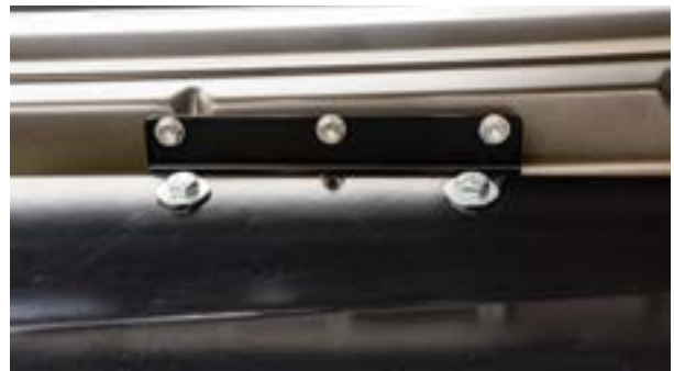
▲ Figure 48. Fully installed door mounting bracket. Looking up from the bottom of the door.
