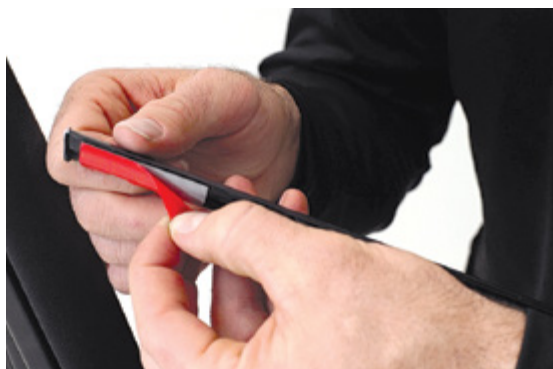
▲ Figure 29. Peeling double-sided adhesive backer
