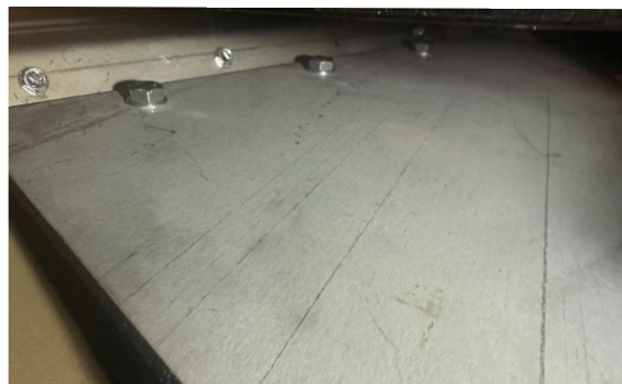
▲ Figure 41. Example of bracket surfaces sitting flush with the interior sheet metal
