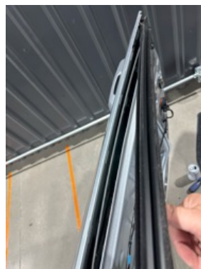
▲ Figure 24. Removing interior window seal
